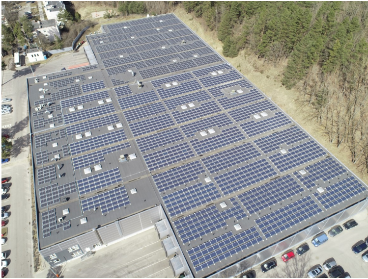
Photo: The solar power plant on the roof of HPP Baltic Sorting Centre in Vilnius.
